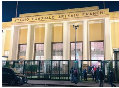
Firenze, Italy. Light Commercial duct and cassette in the restaurant and living areas, RAC in the dressing rooms.
